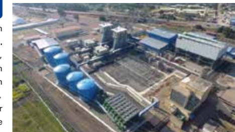
MOZAMBIQUE : EDM MAPUTO POWER PLANT
