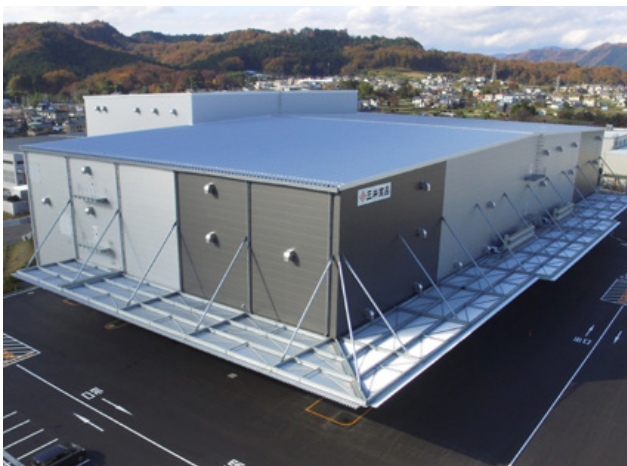
Mitsui Foods Distribution Center
