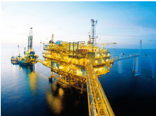
Offshore Thailand gas facilities
