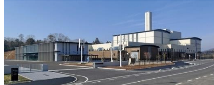
Waste to Energy Plants
