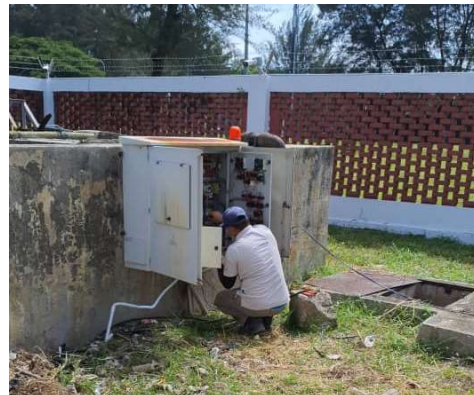
Electrical Construction Work (3 days)
