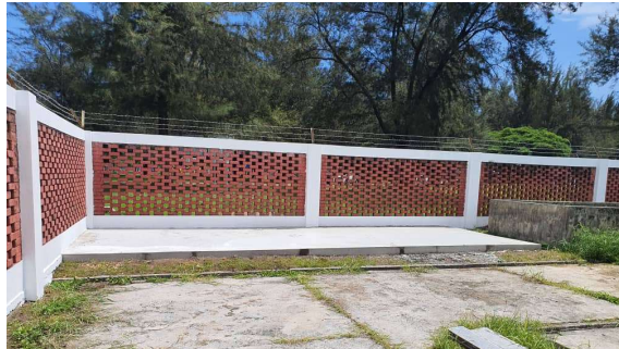
Foundation Construction (2 days)
