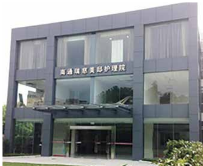
MCS's first nursing care facility (106 beds) in Nantong city, China
