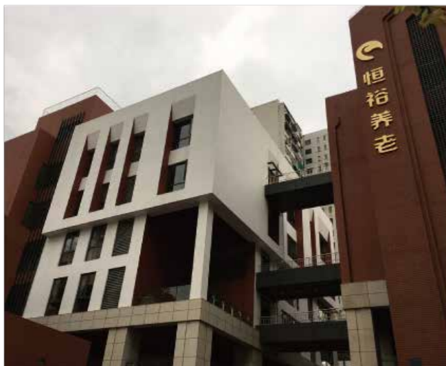
Shanghai Jingan District consulting welfare facility
