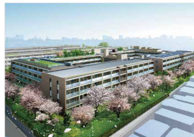
Setagaya Nakamachi Project Condominiums and senior housing
