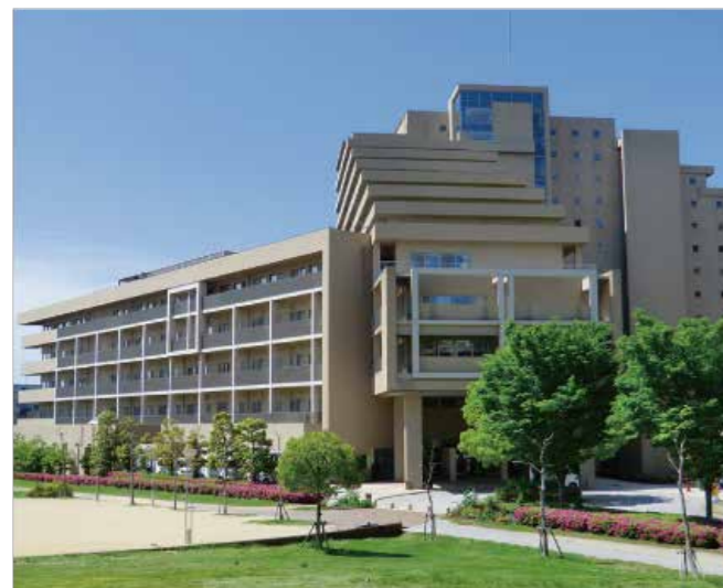
Appearance of the elderly care facilities
