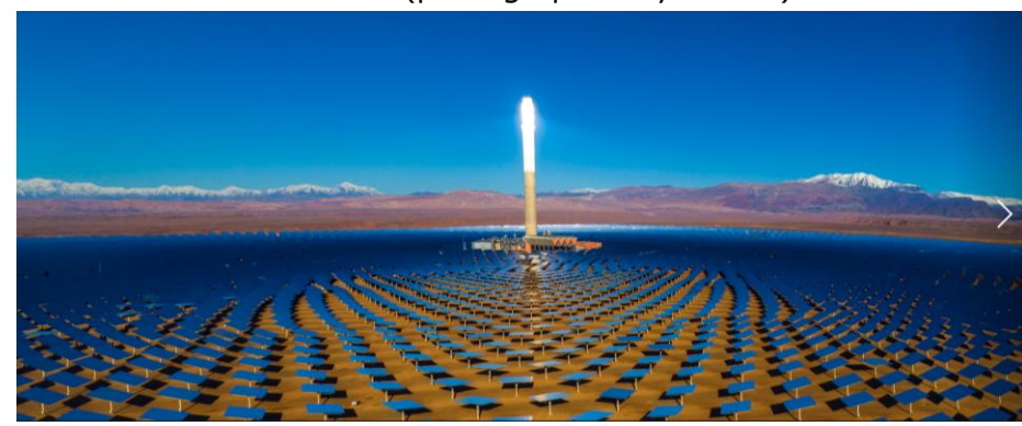
Photovoltaic complex in Morocco (Courtesy of MASEN)
