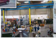
● Torrance plant, U.S.A. MAYEKAWA U.S.A., INC.
