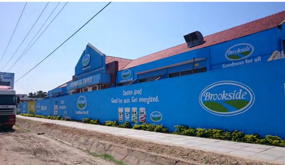
Mombasa DEPO外観
