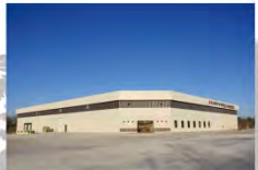
● Nashville Plant Mayekawa U.S.A., Inc.
