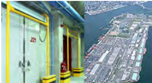
Cold Storage (logistics)
