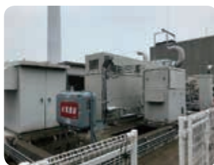
Left: Ammonia mono-fuel combustion micro gas turbine power generation unit with 50kw power output (National Institute of Advanced Industrial Science and Technology)
